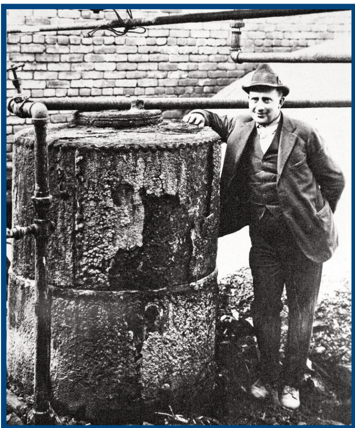
Kier with his Five Barrel Still — A reproduction of a vintage photograph showing Kier (or a representative figure) next to the five barrel still he used to refine petroleum. The original still is preserved at the Drake Well Museum in Titusville, Pa.
