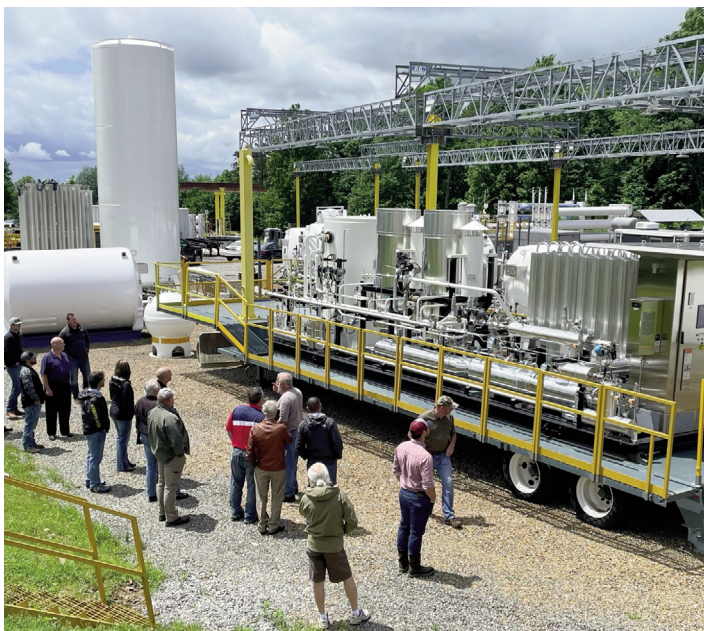
PIOGA Market Development Committee members learn about the trailer-mounted LNG processing unit at Sunnyside Energy Park.
